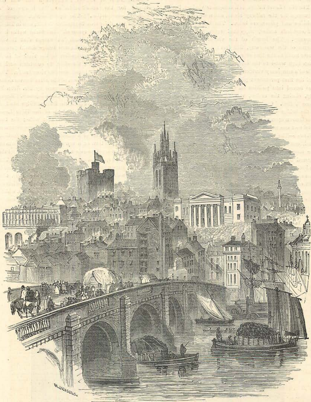
TYNE BRIDGE, NEWCASTLE-ON-TYNE, 1859.
