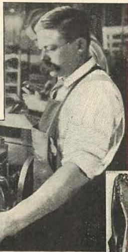
THE LASTING-MACHINE, WHICH STRETCHES THE UPPERS OVER THE LASTS.
