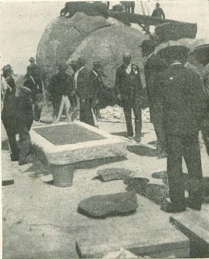
Sealing down the granite slab with cement
