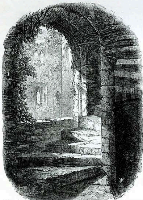
STAIRCASE IN GWENT TOWER.
