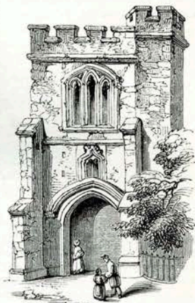
THE CURFEW TOWER, BARKING.
