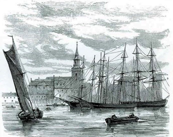
ROTHERHITHE CHURCH: TUNNEL PIER.
