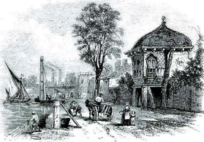
OLD SUMMER-HOUSE AT BATTERSEA.
