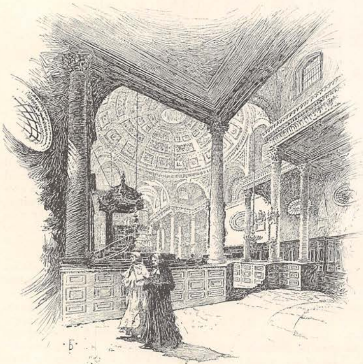
INTERIOR OF ST. STEPHEN, WALBROOK.
