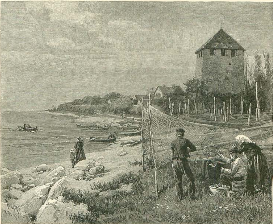
POWDER TOWER AND PART OF THE WALL OF WISBY.
