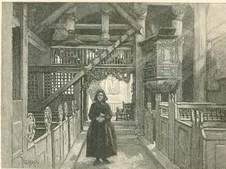
INTERIOR OF OLD CHURCH AT SOGN.
