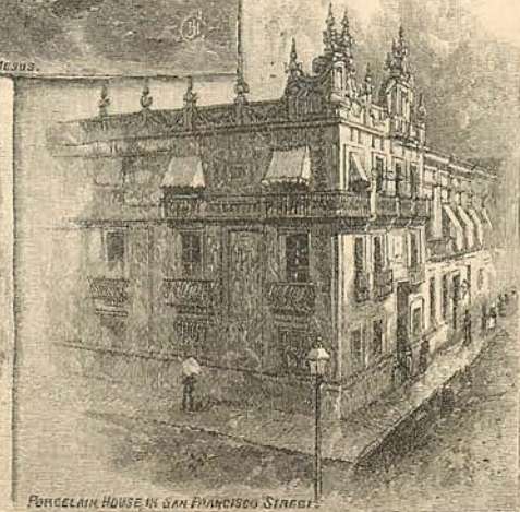
PORCELAIN HOUSE IN SAN FRANCISCO STREET.
