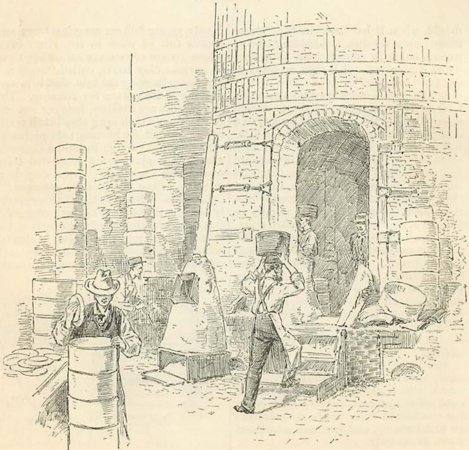
CHARGING A KILN.
