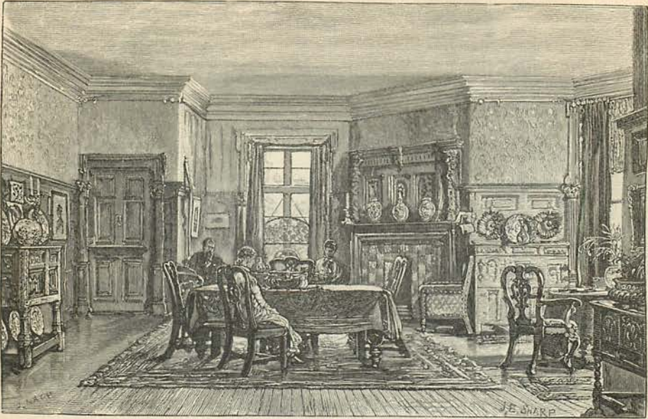
DINING-ROOM IN TOWER HOUSE.
