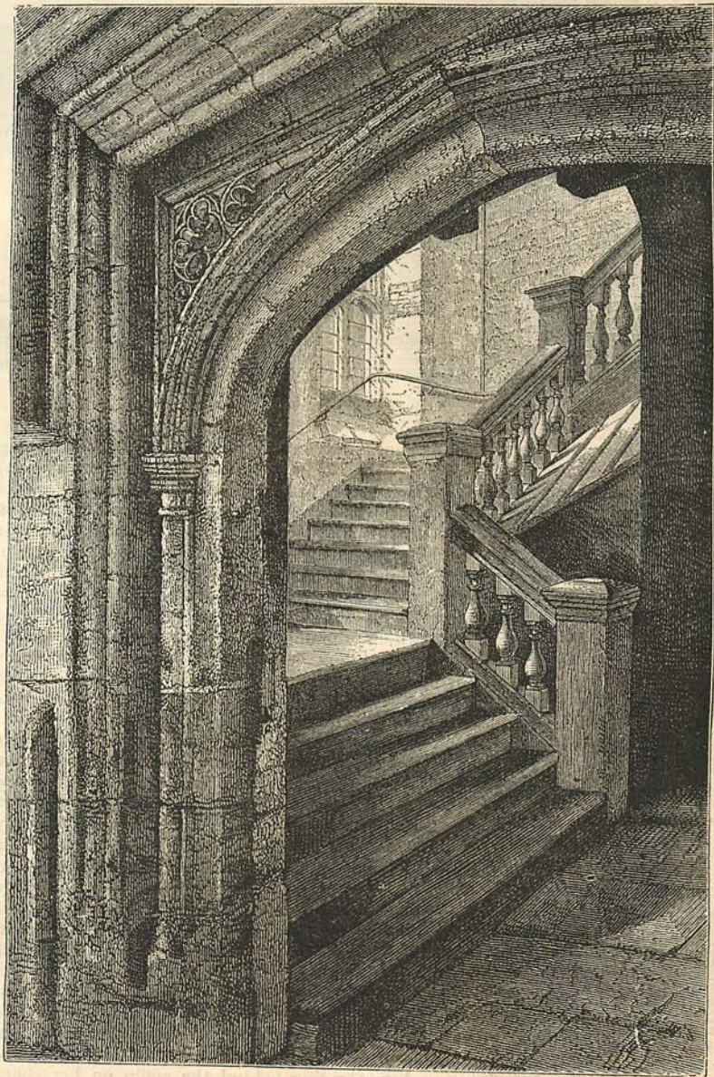
STAIRCASE TO THE CHAPEL AND UPPER SCHOOL.
