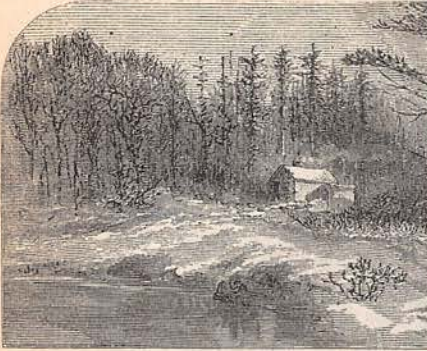
THE TRAPPER'S HUT.
