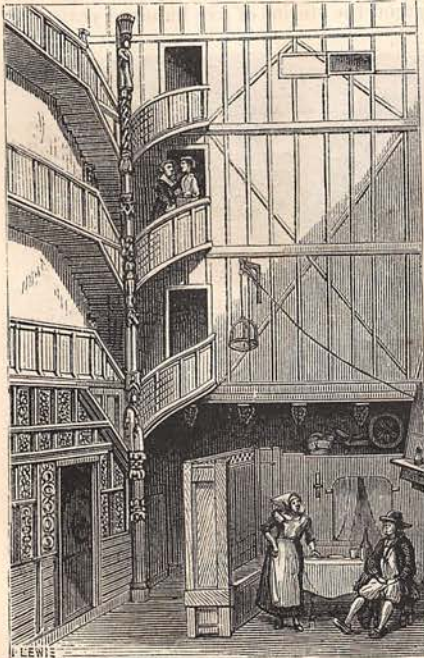
HOUSE INTERIOR, MORLAIX.
