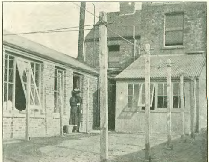
OUTSIDE VIEW OF THE WASH-HOUSE AND BACK OF THE MANAGERESS'S HOUSE.
