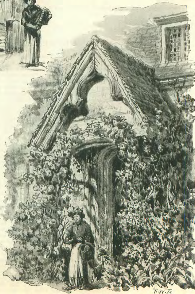
COTTAGE PORCH, PINNER.
