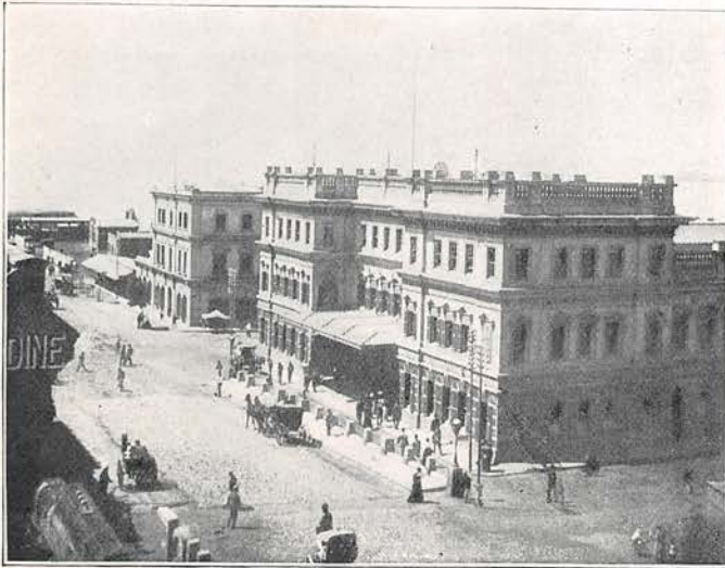
The Beginning of the Great Undertaking: The Railway Station at Cape Town.
