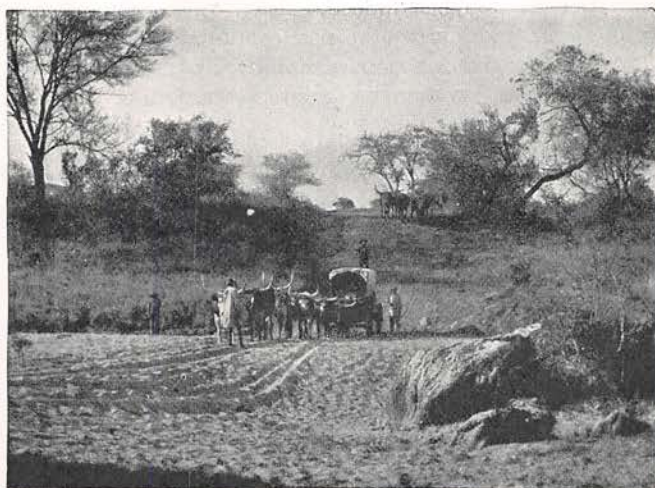
Before the Railway: Crossing a Drift.
