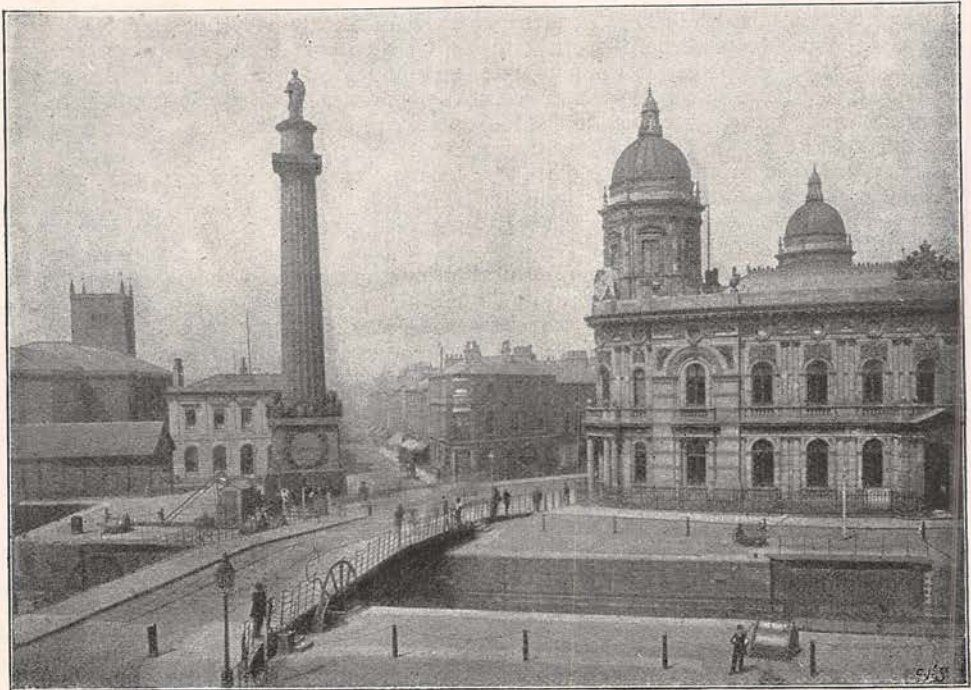
WILBERFORCE MONUMENT AND DOCK OFFICES, HULL.
