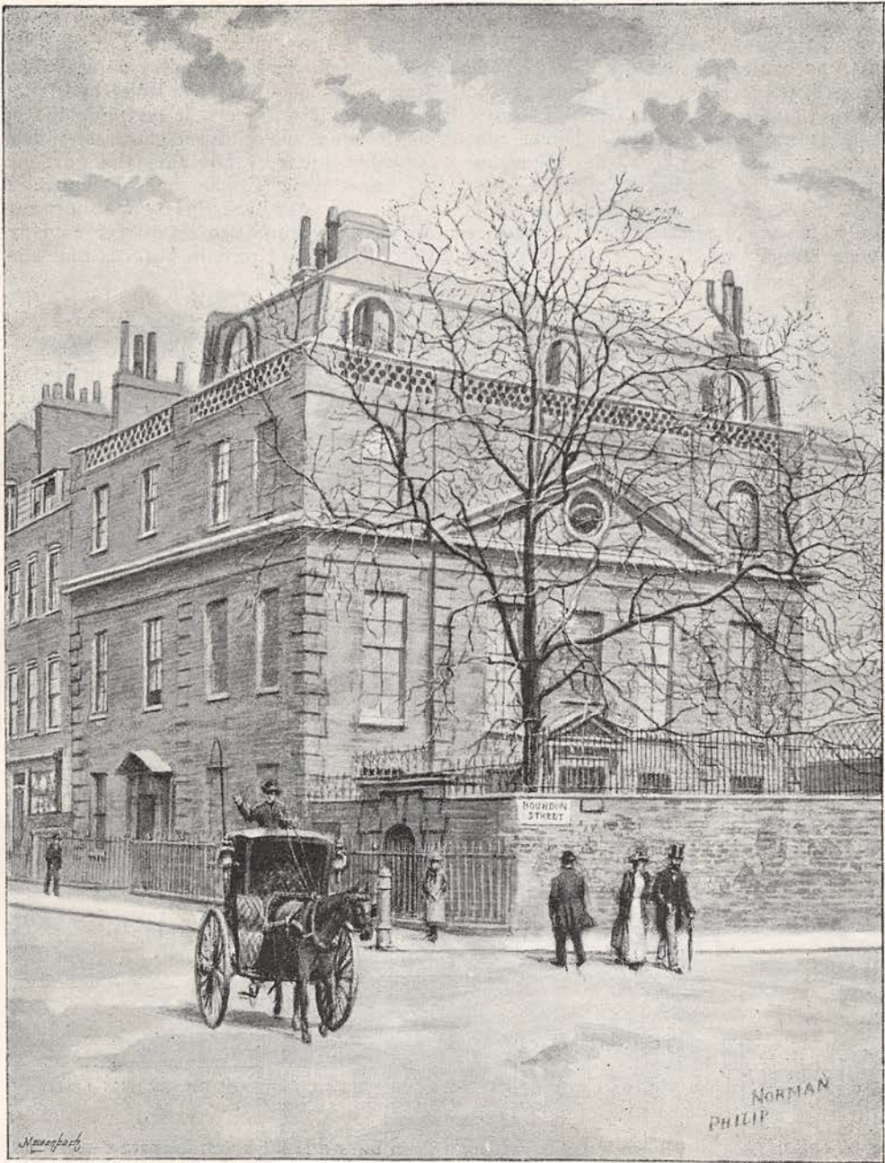
BOURDON HOUSE, DAVIES STREET.
