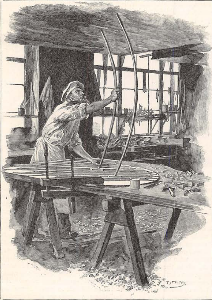
STRENGTHENING A SOUNDING BOARD, USING GOBARS.
