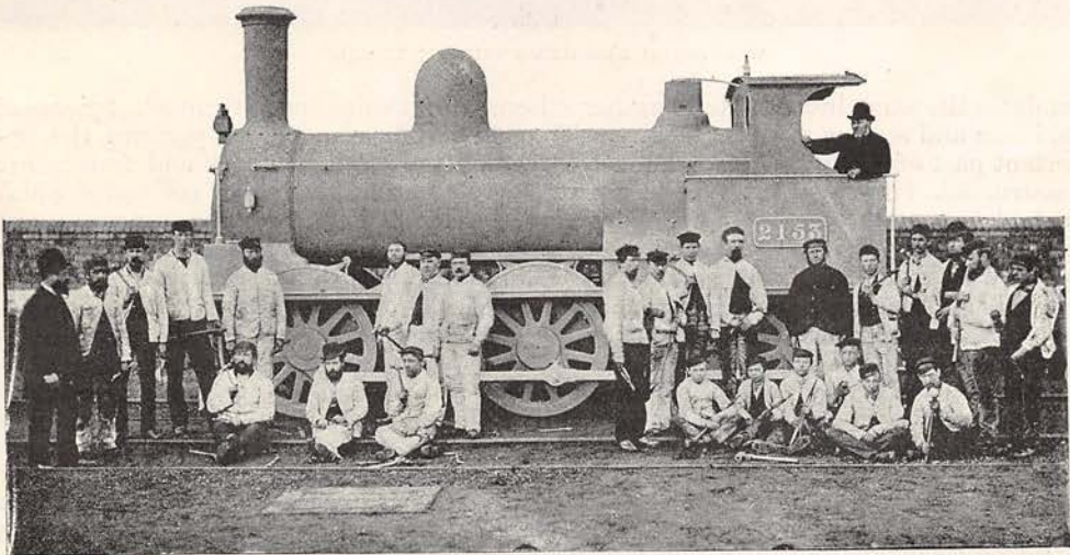
ENGINE ERECTED IN TWENTY-FIVE HOURS AND A HALF. COMPLETED ONE P.M. WEDNESDAY, FEB. 6TH: AND WORKMEN.
