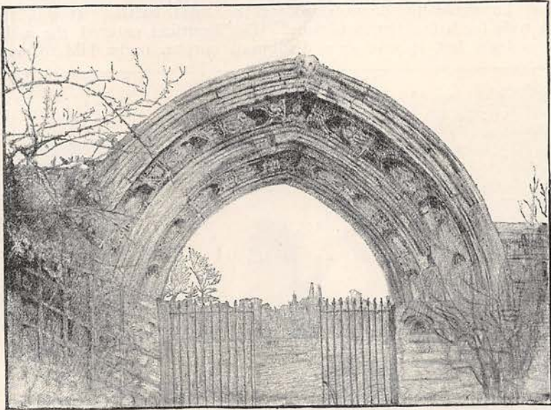
RUINED ARCH-ENTRY TO CHAPTER HOUSE.
