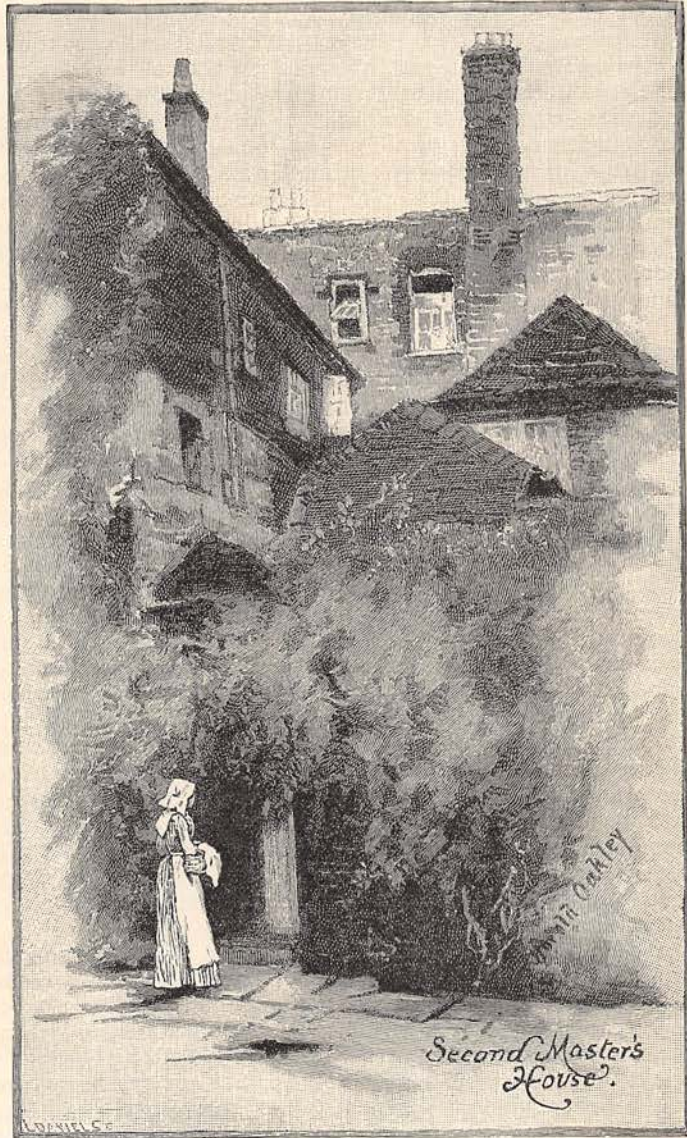
ENTRANCE TO SECOND MASTER'S HOUSE.
