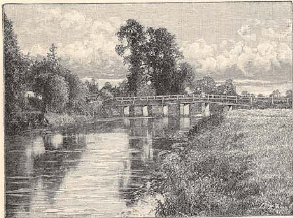
CASTLE EATON BRIDGE.
