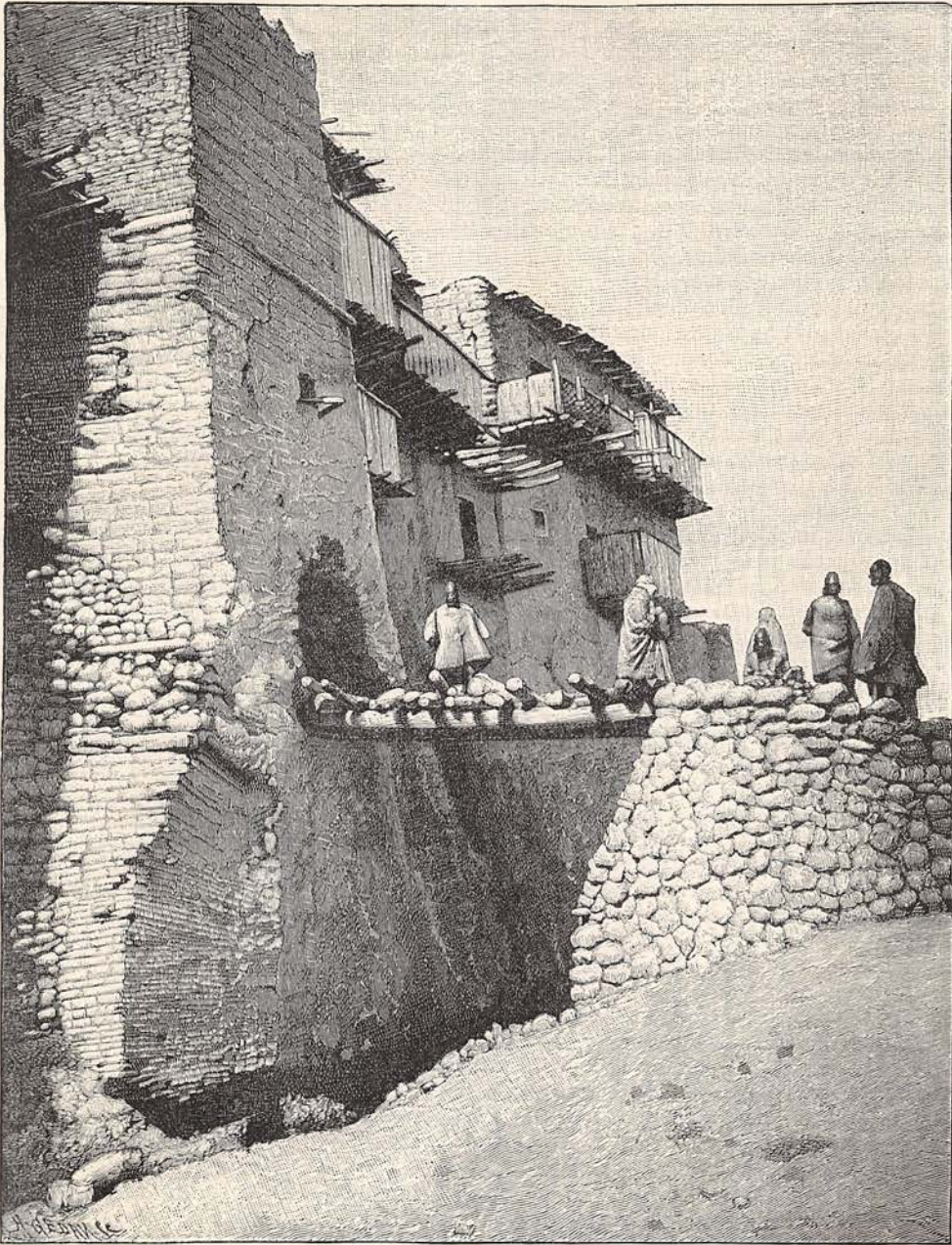
BRIDGE AND ONLY ENTRANCE TO YEZD-I-KHAST.
