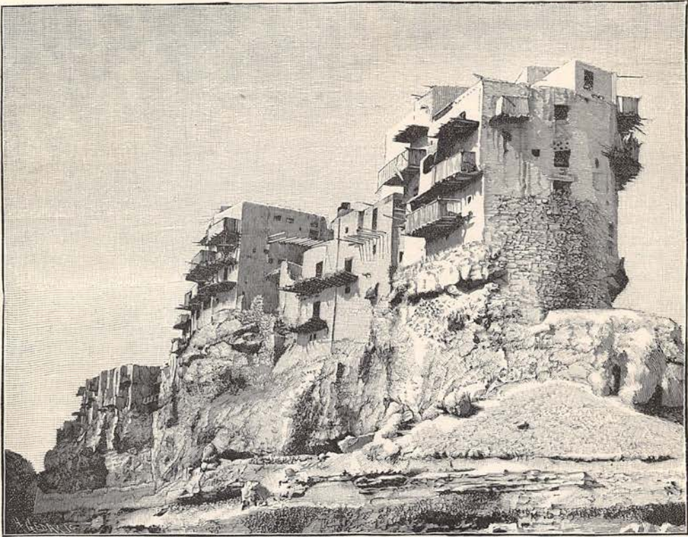
YEZD-I-KHAST FROM THE ROOF OF THE POST-HOUSE.
