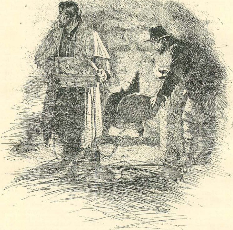
WORKING AT THE TUNNEL.
