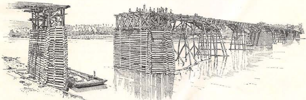
MILITARY BRIDGE OVER THE TENNESSEE RIVER AT CHATTANOOGA, BUILT BY THE UNITED STATES ENGINEERS IN OCTOBER, 1863, JUST AFTER THE BATTLE OF CHICKAMAUGA. (FROM A PHOTOGRAPH BY R. M. CRESSEY, LENT BY GENERAL G. P. THRUSTON.)
