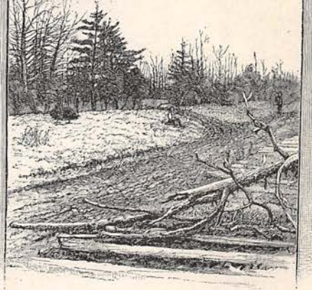
THE PLANK-ROAD NEAR WHERE JACKSON FELL.
