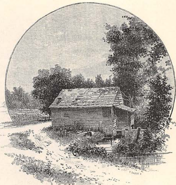
ROWLETT'S MILL, ON THE EDDYVILLE ROAD AT HICKMAN'S CREEK.
