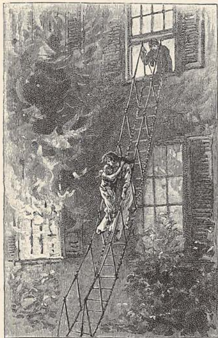
THE NEW FIRE-ESCAPE IN USE.
