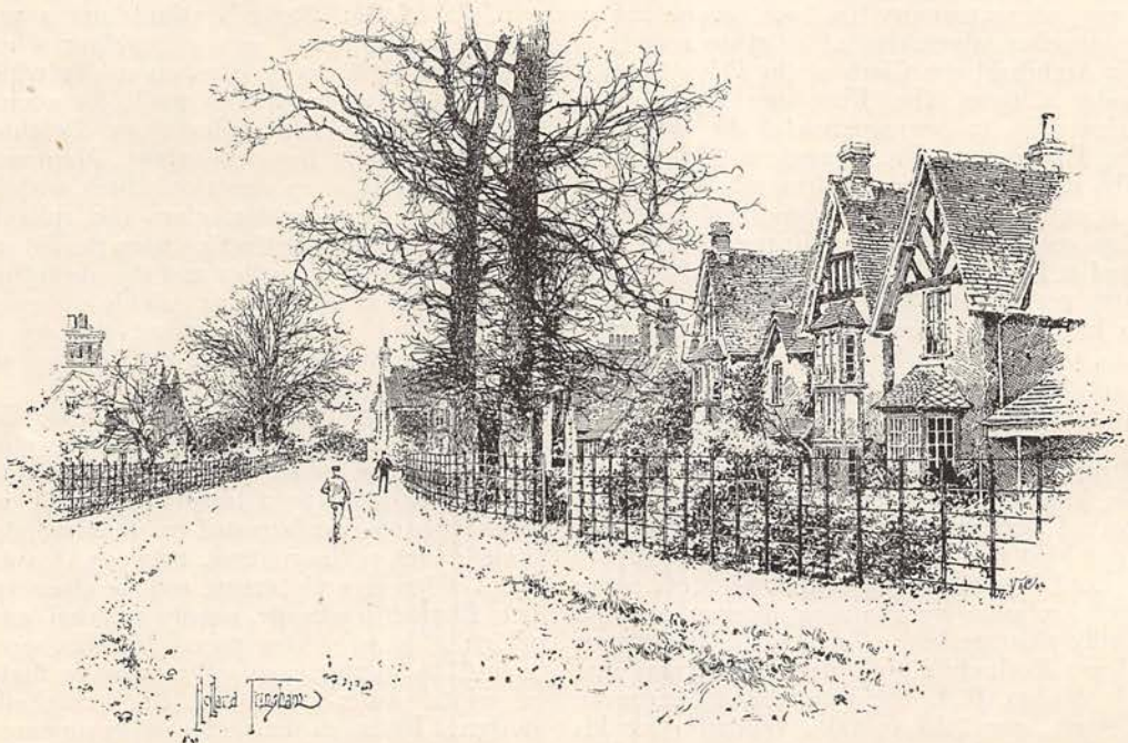
MENTMORE VILLAGE.—COTTAGES BUILT BY LADY ROSEBERY.
