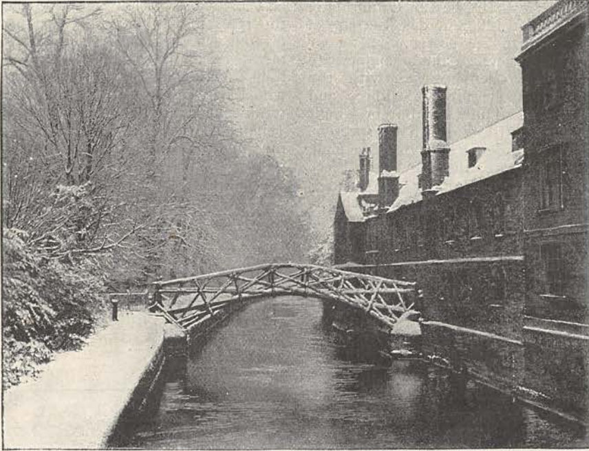
QUEEN'S COLLEGE BRIDGE.
