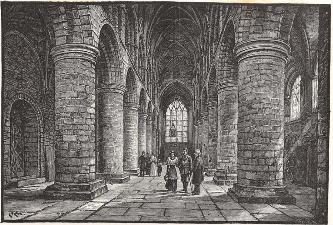
THE NAVE, KIRKWALL CATHEDRAL, LOOKING EAST.
