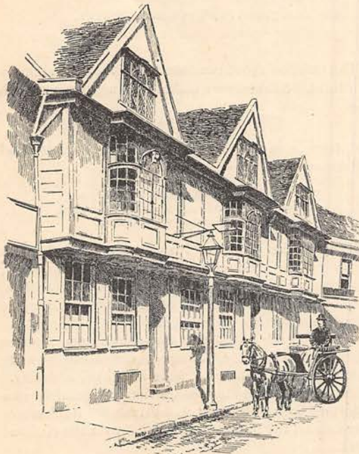
OLD HOUSES, FORE STREET.
