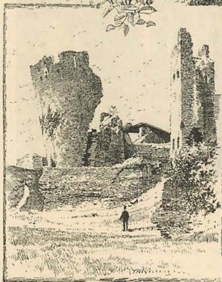
LEANING TOWER, CAERPHILLY.
