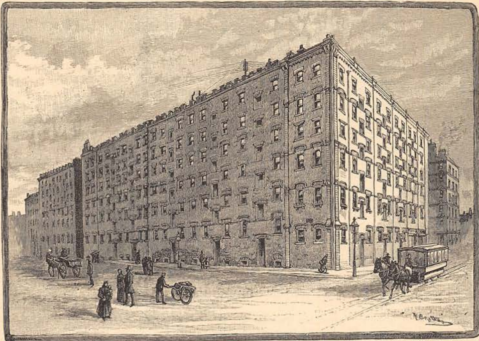
QUEEN'S BUILDINGS, SOUTHWARK BRIDGE ROAD. (On the Site of the Old Queen's Bench Prison.)
