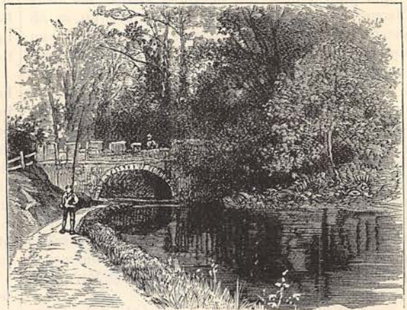
BRIDGE ON CANAL.
