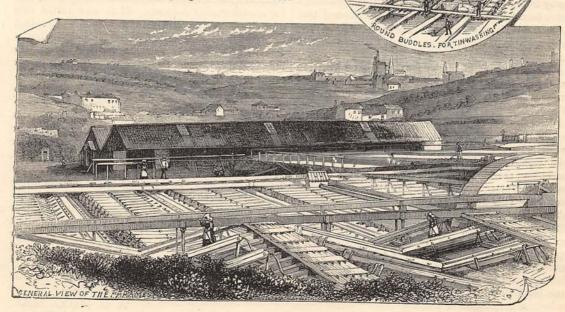
of water-power, too intricate to be here described. The fluid flows on to the top of one frame, trickles down its surface, is received in a shoot at the bottom and thence transferred to the next. At regular intervals, the supply being cut off, there is left behind on the frame a thin coat of tin-dust. A stream of clean water now emptied over the frame with some force washes the dust down with it into a receiver
