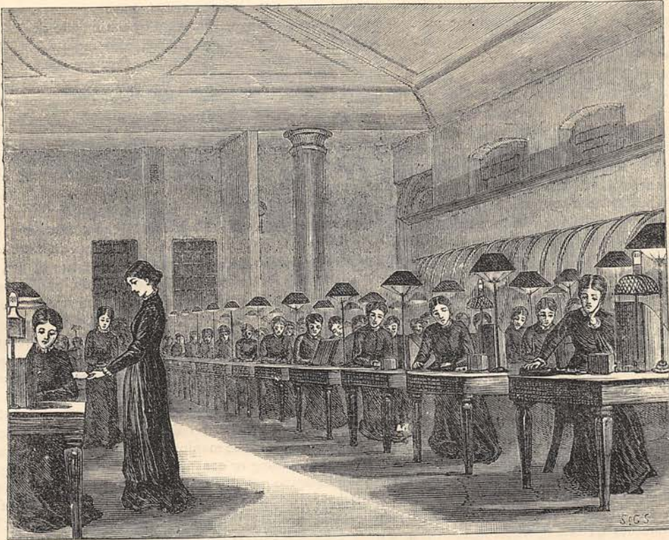
THE OPERATING ROOM AT THE GENERAL POST OFFICE.
