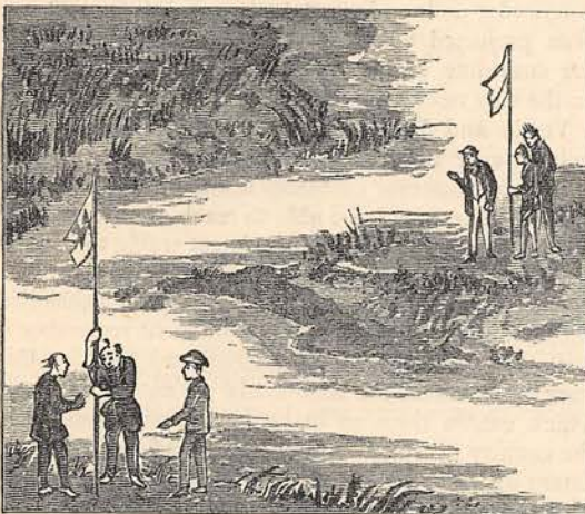
SURVEYING FOR A NEW RAILWAY (from an original Japanese Drawing)
