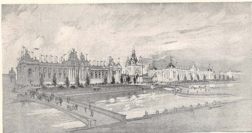
AGRICULTURE, ADMINISTRATION, AND MINES BUILDINGS.
