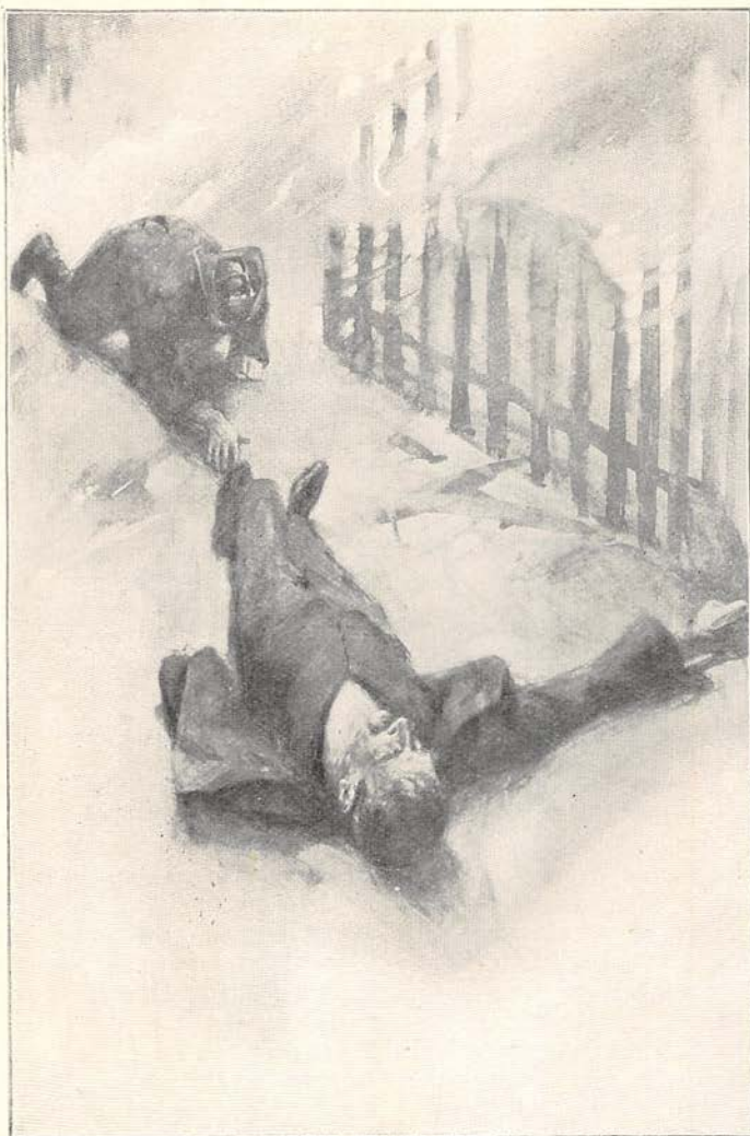
FOREMAN AHEARN RESCUING THE INJURED PUMPER DEVOE OVER TANKS OF NAPHTHA.
