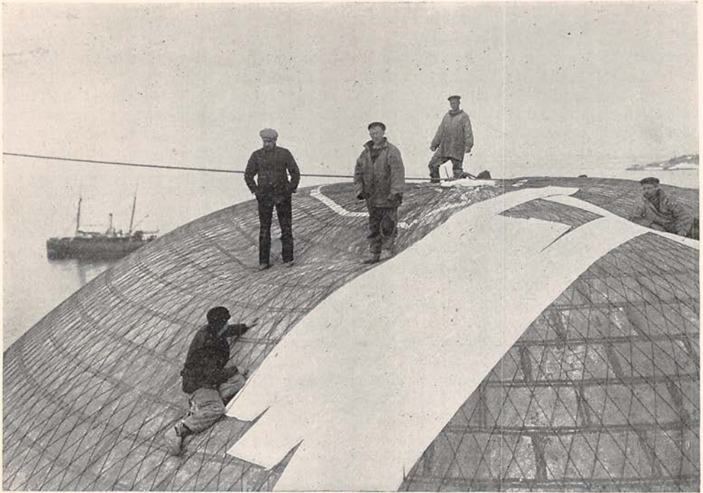
SEARCHING FOR LEAKS WITH CLOTH PREPARED WITH CHEMICALS.
