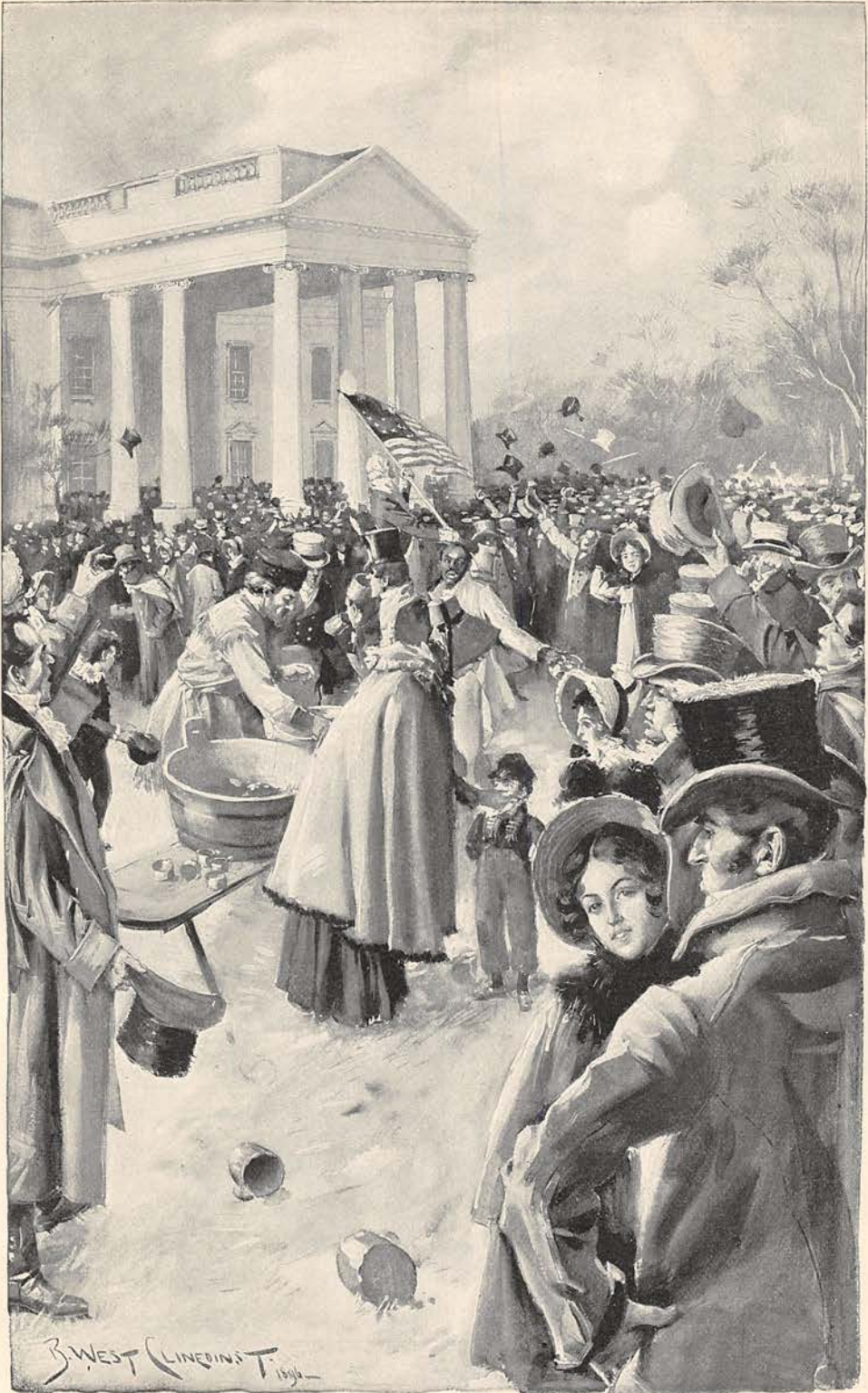
THE CRUSH AT THE WHITE HOUSE AFTER JACKSON'S INAUGURATION.
