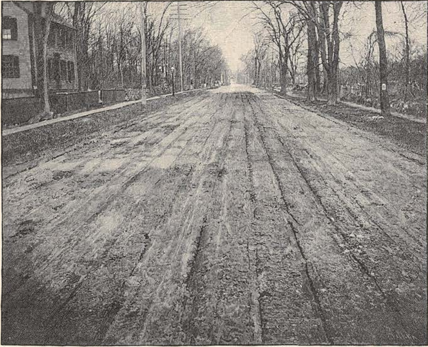
VIEW OF BLUE HILL AVENUE, MATTAPAN, MASSACHUSETTS.
