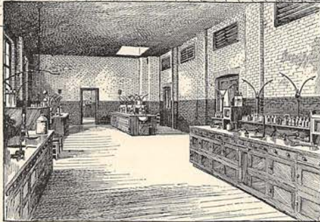
MACHINE SHOP, GYMNASIUM, AND CHEMICAL LABORATORY, PEOPLE'S PALACE.
