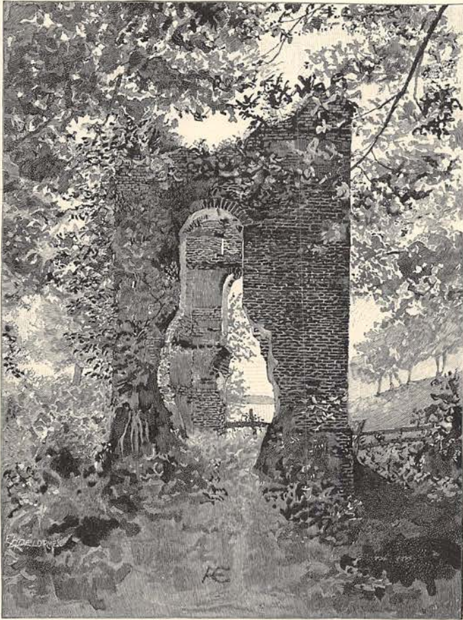
OLD CHURCH TOWER, JAMESTOWN.
