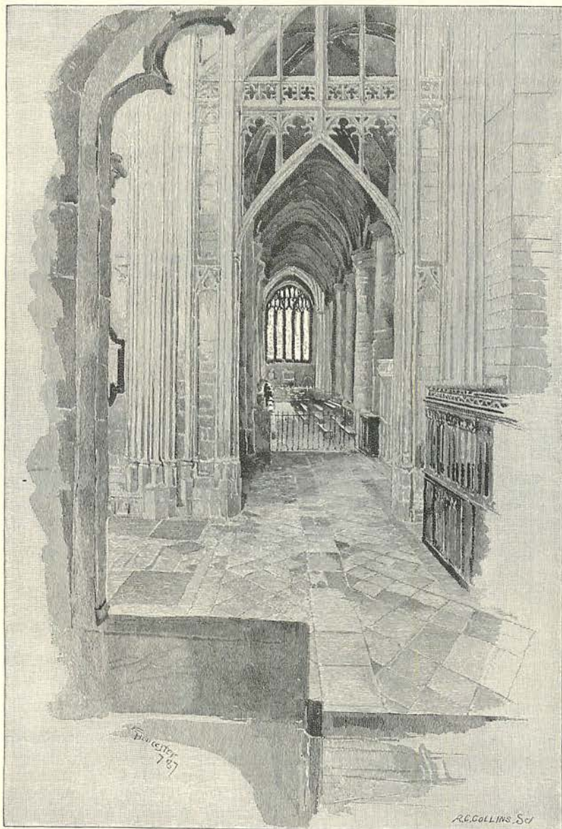
SOUTH AISLE OF THE NAVE, LOOKING WEST FROM THE TRANSEPT.
