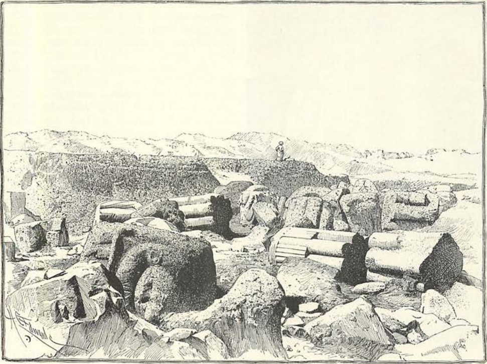
VIEW OVER THE RUINS OF THE HYPOSTYLE HALL.
