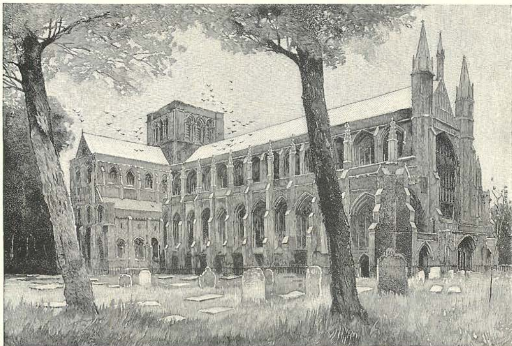
THE NAVE OF WINCHESTER.
